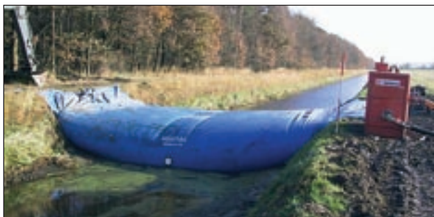
Canal Repair Hoogeveen, Netherlands
