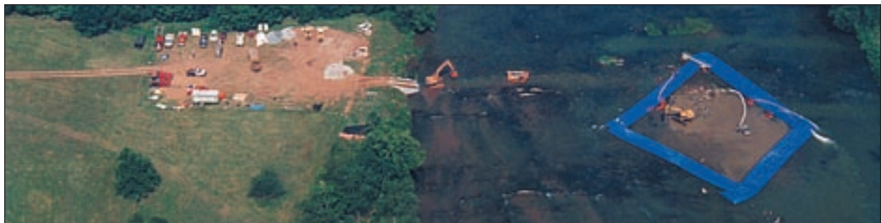
Staunton River, Brookneal, VA Pipeline Repair
