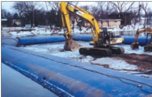
Fox River, Burlington, WI Pipeline Installation 425 linear feet of 6-ft barriers installed in 11 hours.
