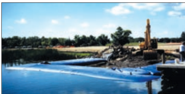
Lake of the Woods, Warroad, MN. Boat Ramp Installation
